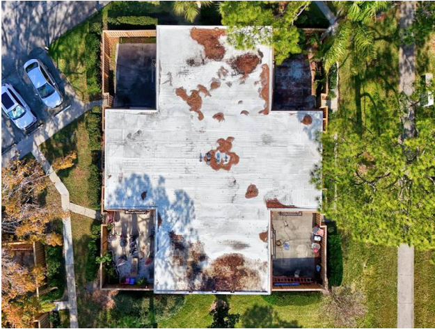
ROOF - CONCRETE WITH TPO COVERING
