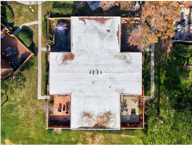
ROOF - CONCRETE WITH TPO COVERING
