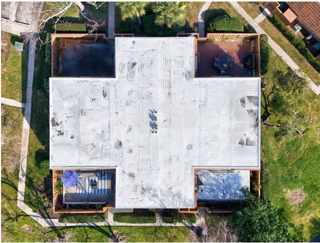
ROOF - CONCRETE WITH TPO COVERING
