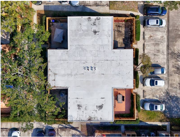
ROOF - CONCRETE WITH TPO COVERING
