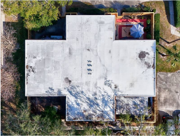
ROOF - CONCRETE WITH TPO COVERING
