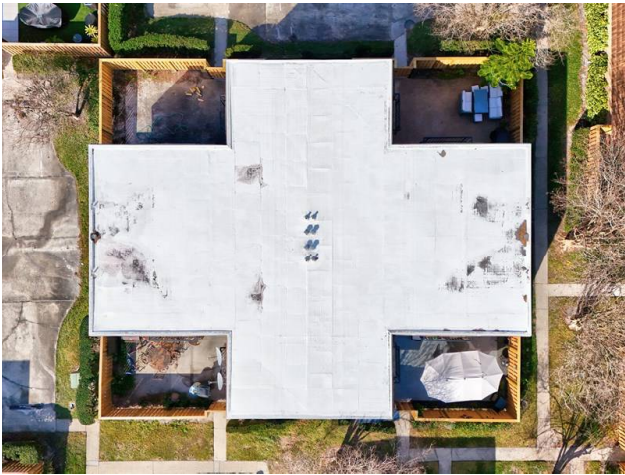
ROOF - CONCRETE WITH TPO COVERING
