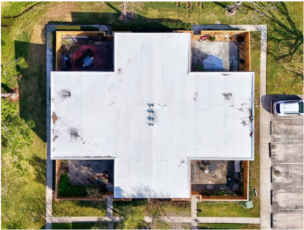
ROOF - CONCRETE WITH TPO COVERING
