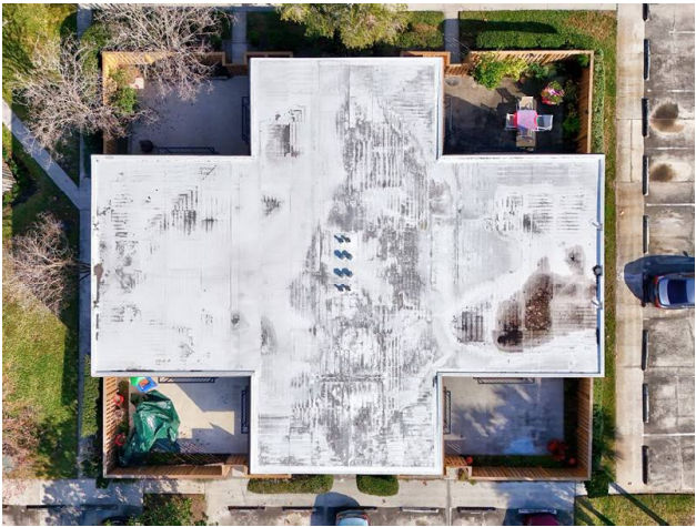
ROOF - CONCRETE WITH TPO COVERING
