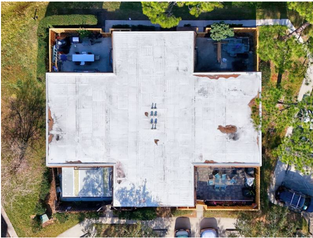
ROOF - CONCRETE WITH TPO COVERING
