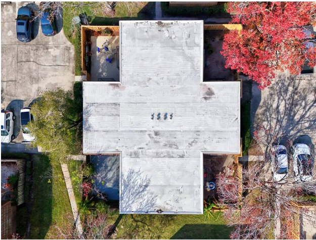
ROOF - CONCRETE WITH TPO COVERING
