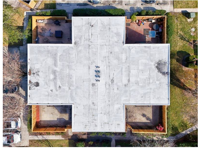
ROOF - CONCRETE WITH TPO COVERING
