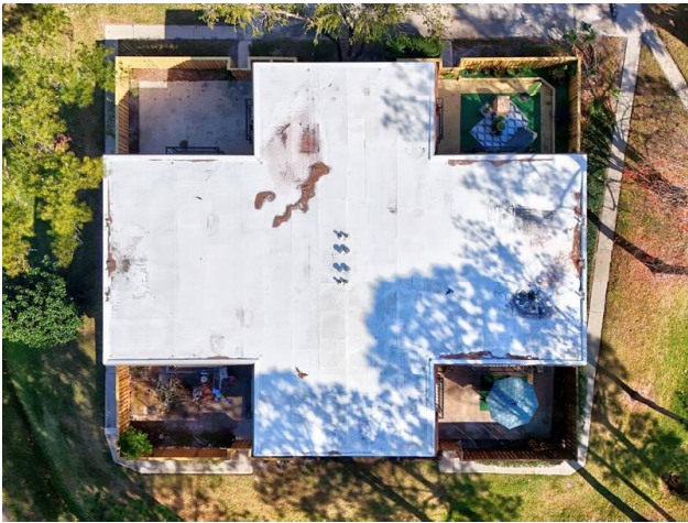
ROOF - CONCRETE WITH TPO COVERING
