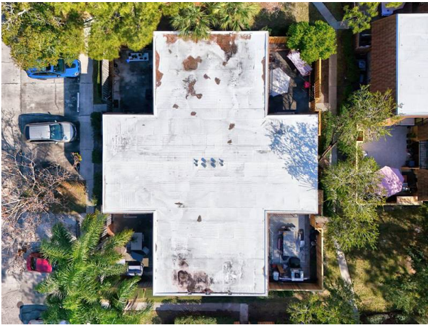
ROOF - CONCRETE WITH TPO COVERING
