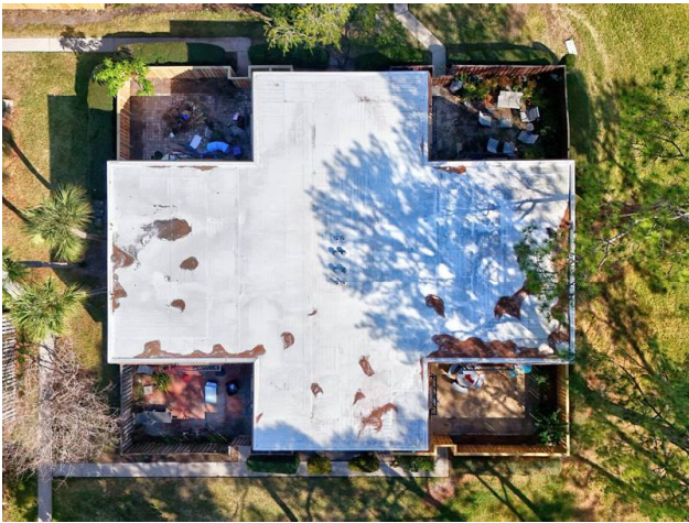
ROOF - CONCRETE WITH TPO COVERING
