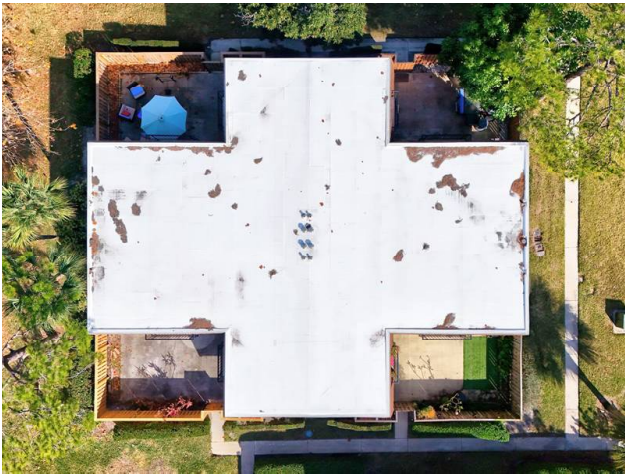
ROOF - CONCRETE WITH TPO COVERING
