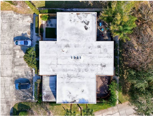
ROOF - CONCRETE WITH TPO COVERING
