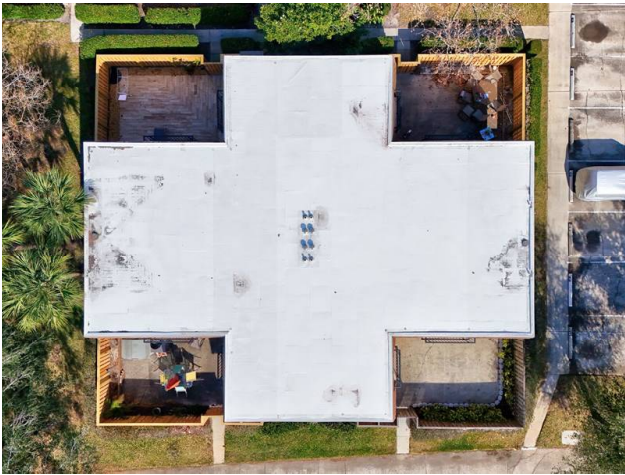
ROOF - CONCRETE WITH TPO COVERING
