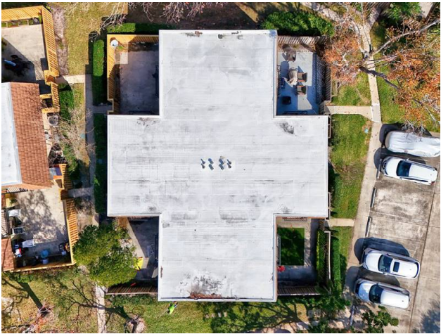
ROOF - CONCRETE WITH TPO COVERING
