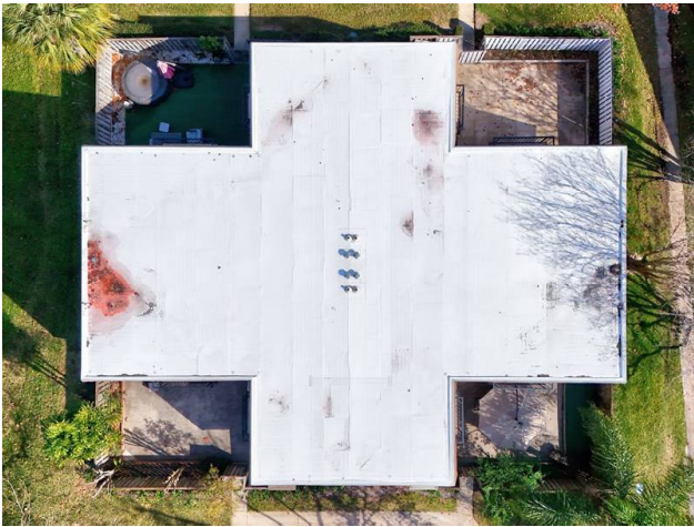
ROOF - CONCRETE WITH TPO COVERING
