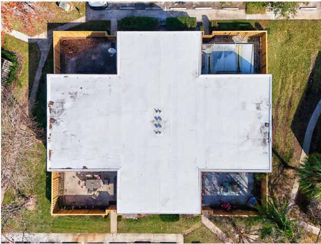
ROOF - CONCRETE WITH TPO COVERING
