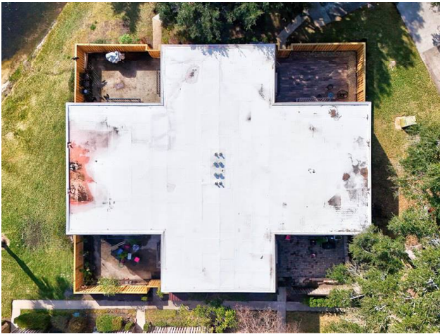
ROOF - CONCRETE WITH TPO COVERING
