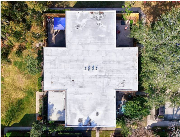
ROOF - CONCRETE WITH TPO COVERING
