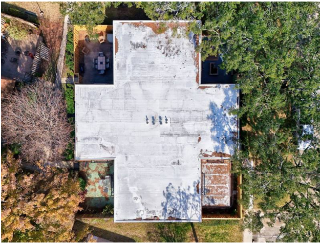
ROOF - CONCRETE WITH TPO COVERING
