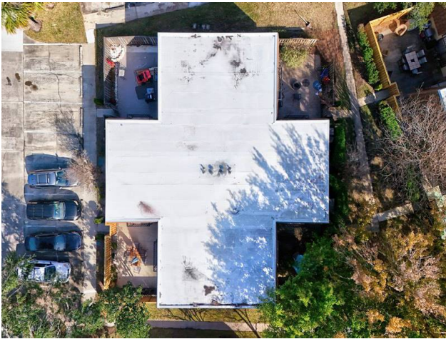
ROOF - CONCRETE WITH TPO COVERING
