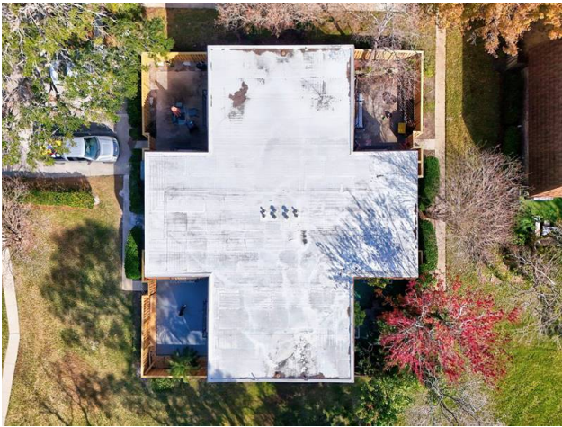
ROOF - CONCRETE WITH TPO COVERING
