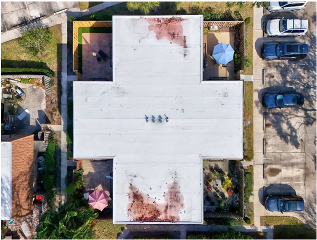
ROOF - CONCRETE WITH TPO COVERING
