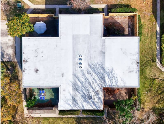
ROOF - CONCRETE WITH TPO COVERING
