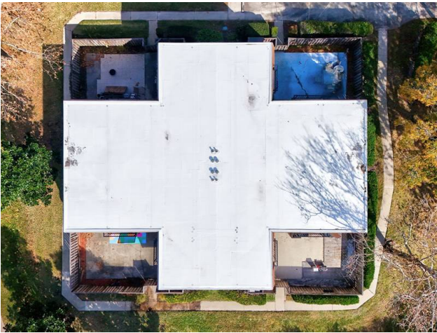
ROOF - CONCRETE WITH TPO COVERING
