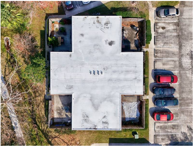
ROOF - CONCRETE WITH TPO COVERING
