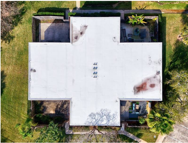
ROOF - CONCRETE WITH TPO COVERING
