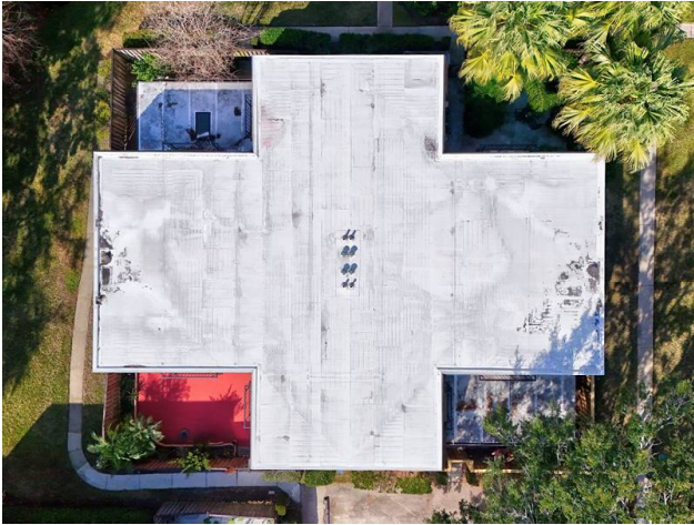
ROOF - CONCRETE WITH TPO COVERING
