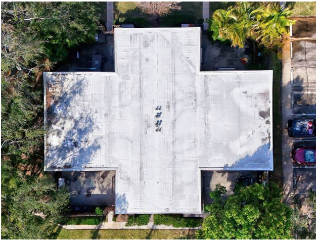
ROOF - CONCRETE WITH TPO COVERING
