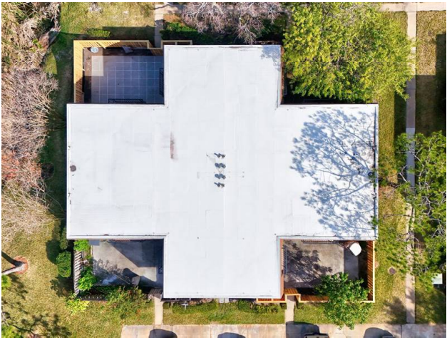
ROOF - CONCRETE WITH TPO COVERING
