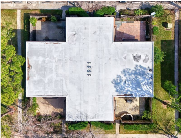
ROOF - CONCRETE WITH TPO COVERING
