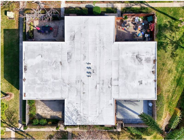
ROOF - CONCRETE WITH TPO COVERING
