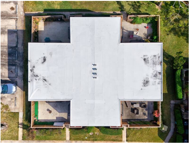
ROOF - CONCRETE WITH TPO COVERING
