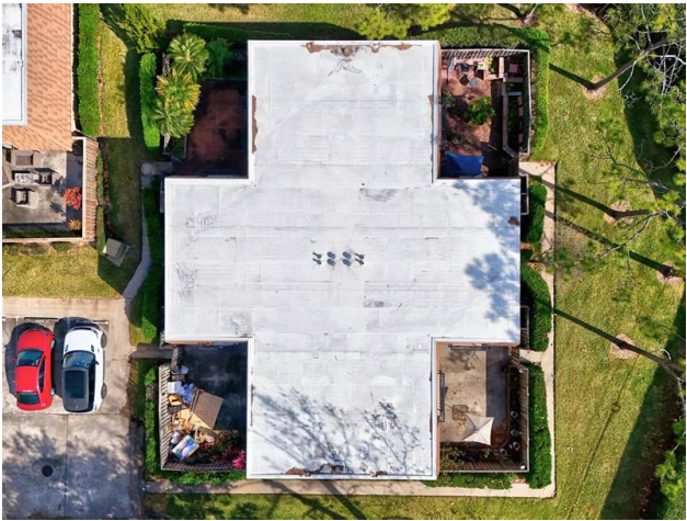
ROOF - CONCRETE WITH TPO COVERING
