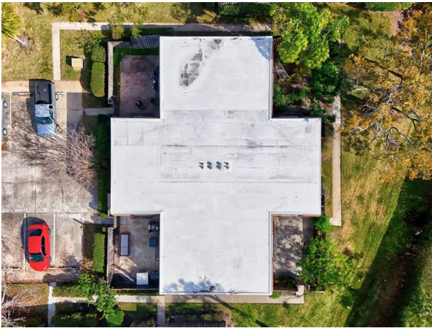
ROOF - CONCRETE WITH TPO COVERING
