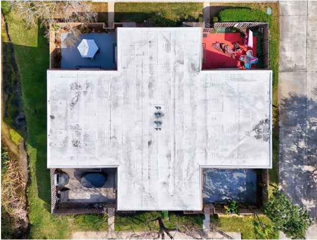
ROOF - CONCRETE WITH TPO COVERING
