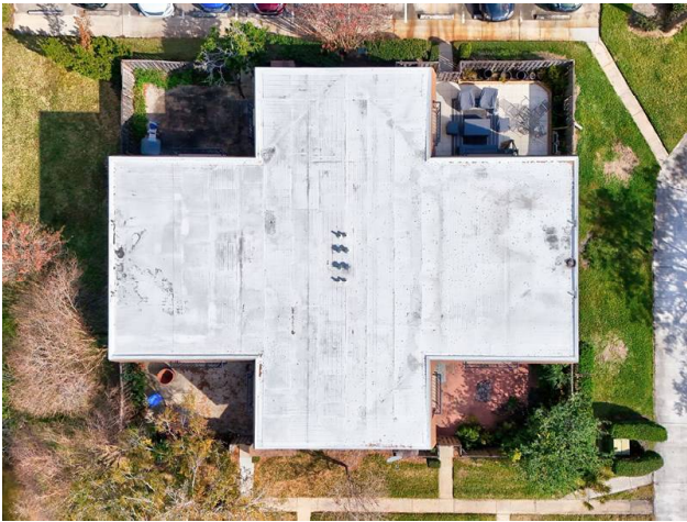
ROOF - CONCRETE WITH TPO COVERING
