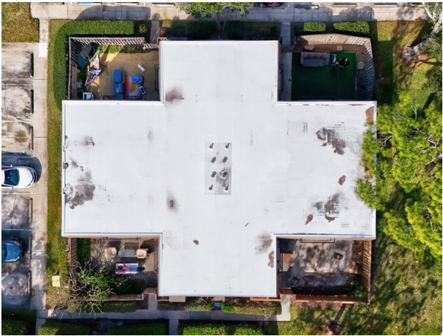
ROOF - CONCRETE WITH TPO COVERING
