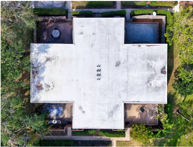
ROOF - CONCRETE WITH TPO COVERING
