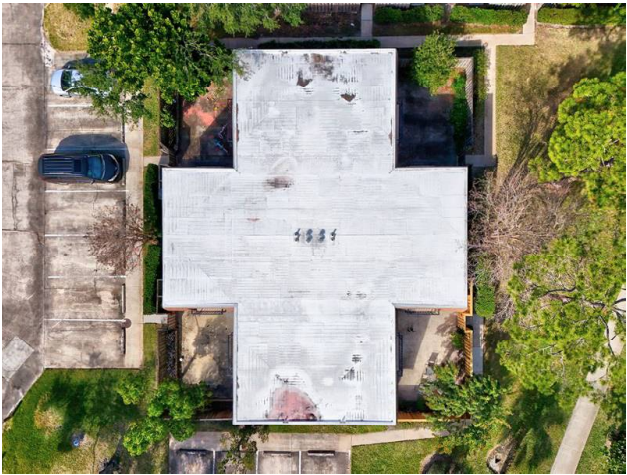
ROOF - CONCRETE WITH TPO COVERING
